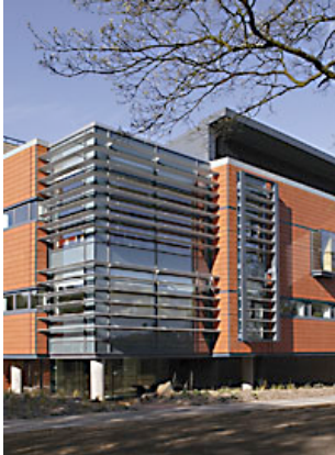
Erskine Williamson Building, University of Edinburgh
